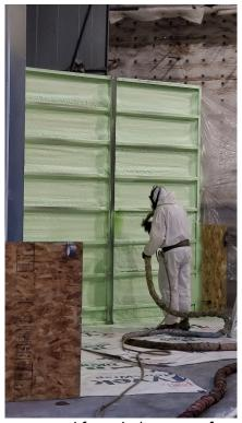
Figure 3: The exposed face during spray foam application.
