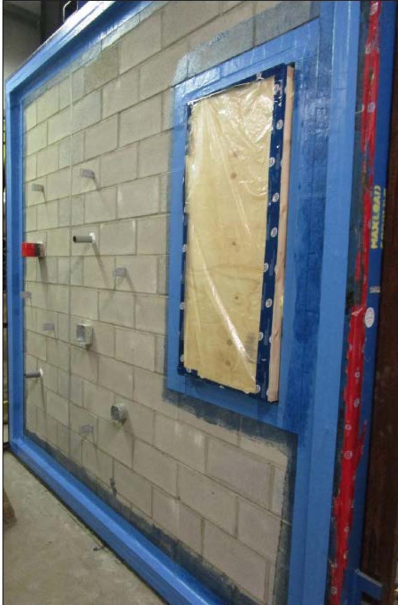
Photo K2 – Penetrations wall section; wall perimeter and window rough open prepared with membrane and penetrations sealed with sealant prior to product application
