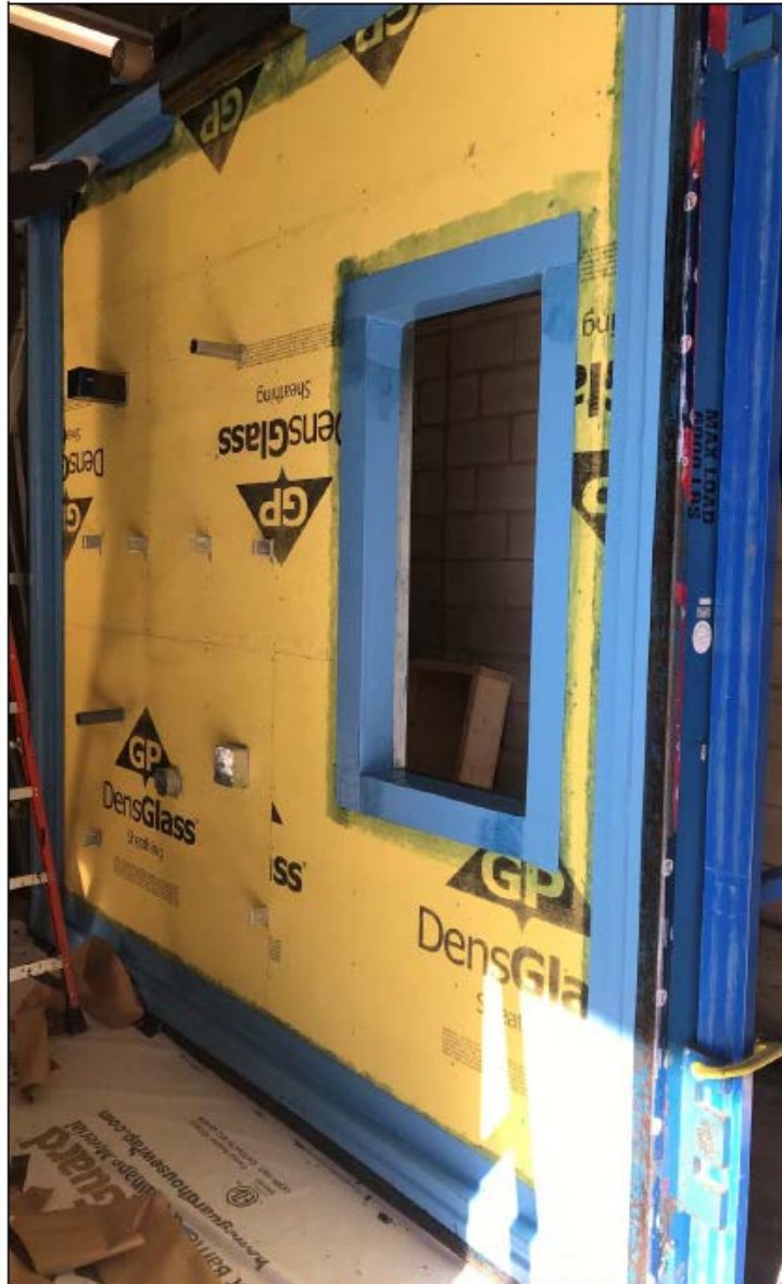
Photo H1 – Penetrations wall section; wall perimeter and window rough open prepared with membrane and penetrations sealed with sealant prior to product application
