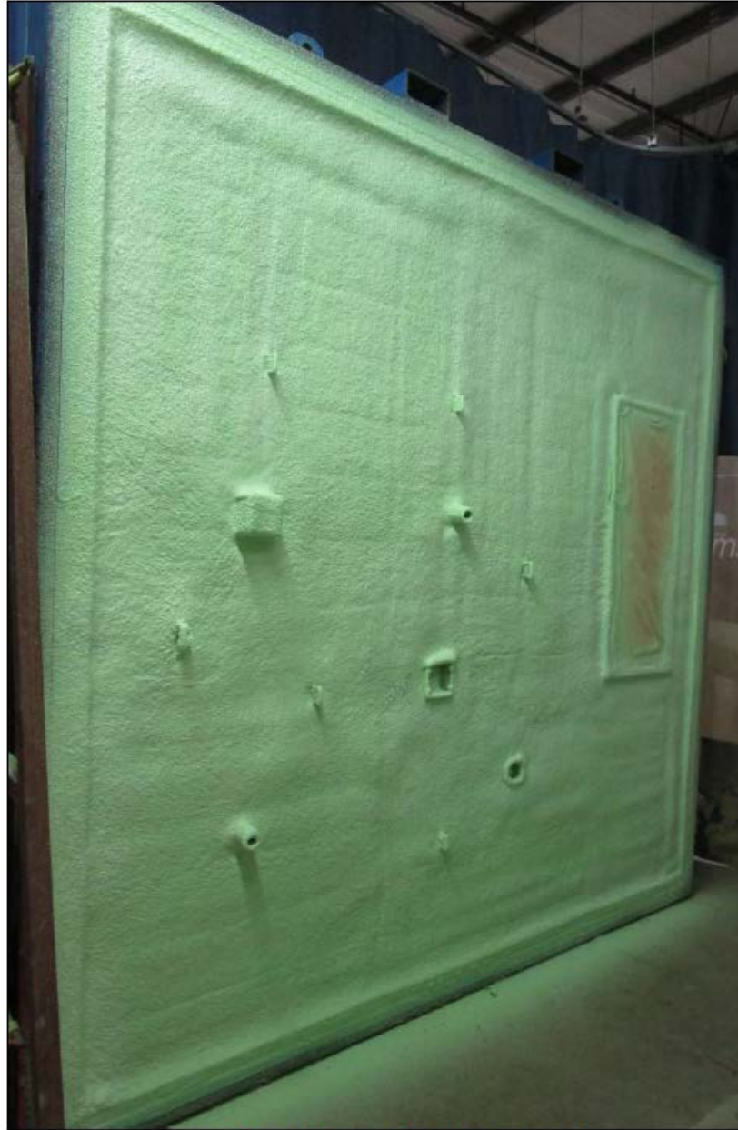
Photo K4 – Air barrier applied onto CMU wall
