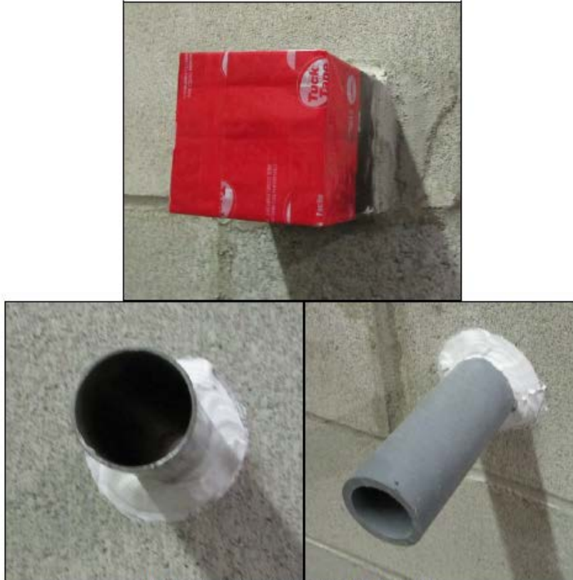
Photo K3 – Penetrations sealed with sealant
