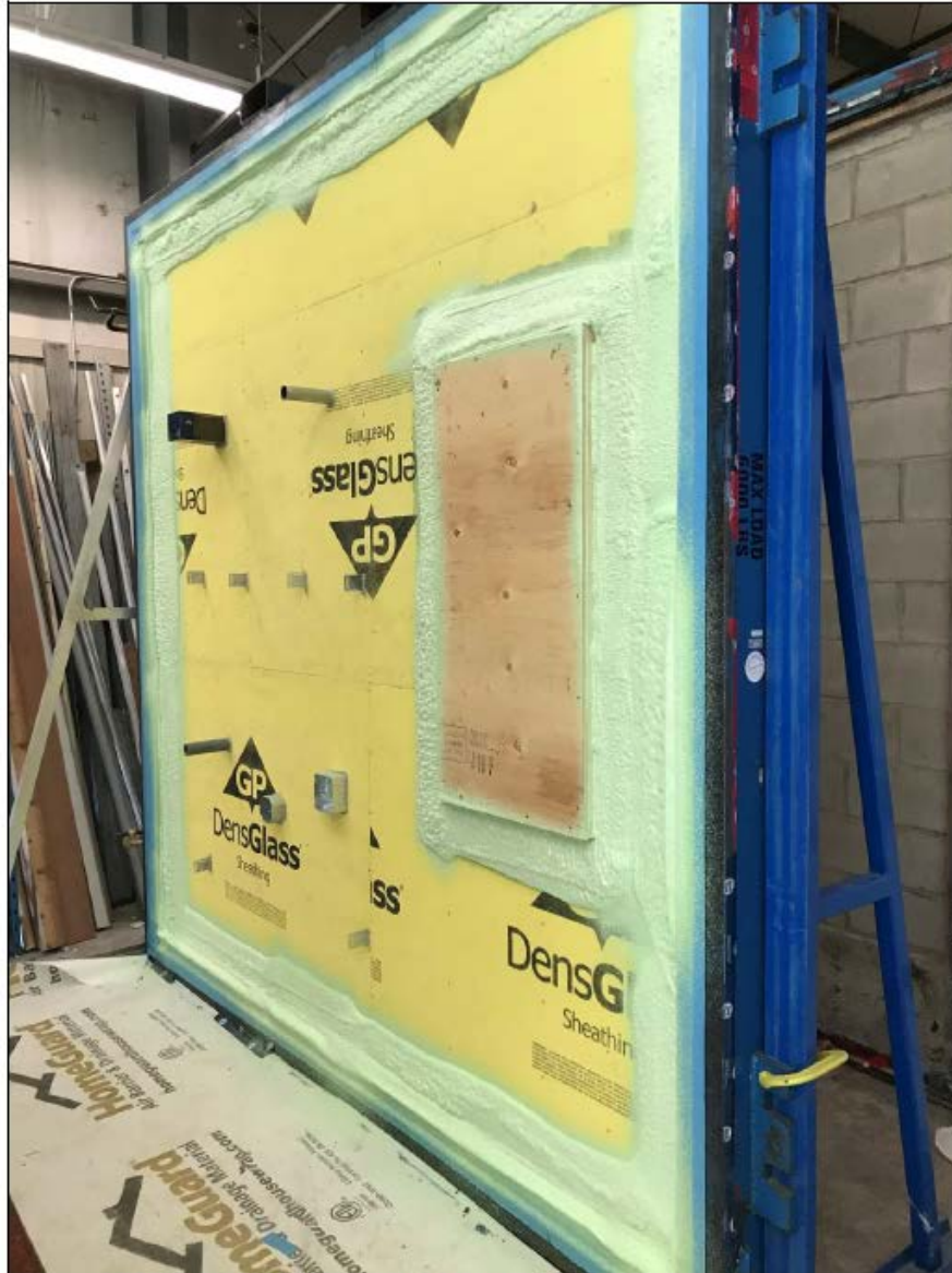
Photo H3 – Air barrier sprayed around wall perimeter and window perimeter
