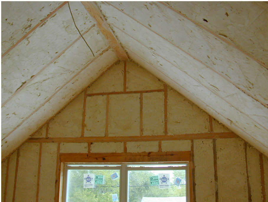
Photograph 2: Spray Foam Insulation
