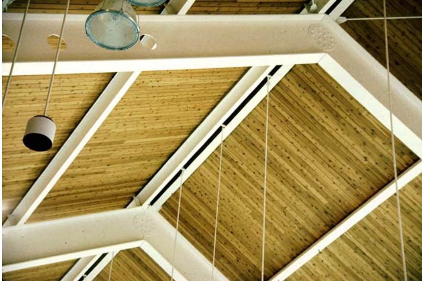
Photograph 4: Compact Roof For Pool Enclosure
