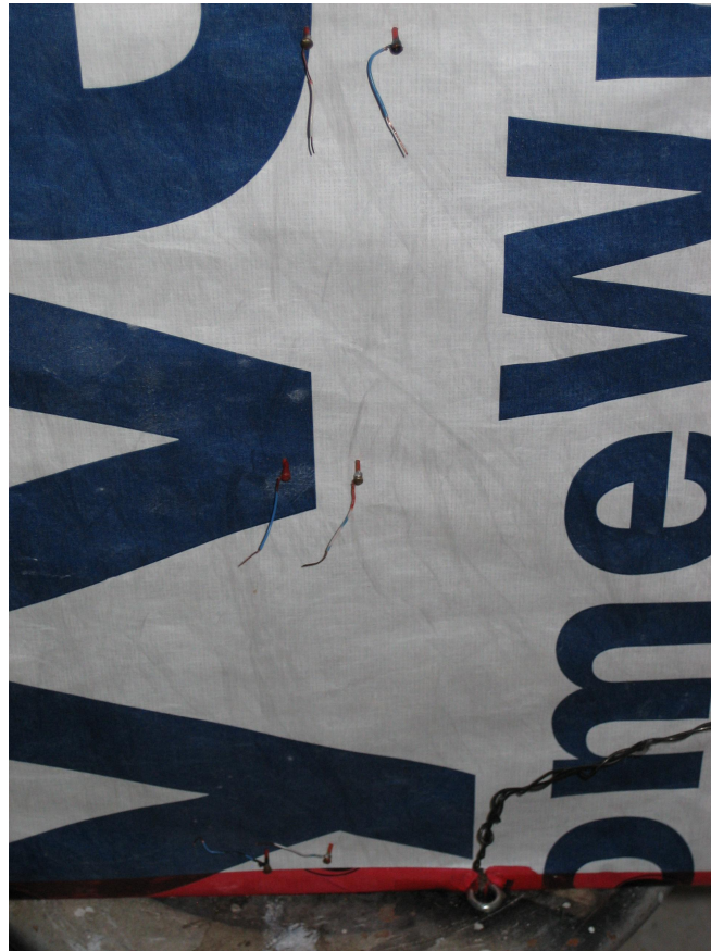
Figure 3.5: Three Moisture Content Pins Installed in Test Panel OSB through Tyvek
