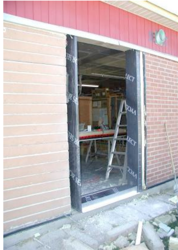
Figure 2.2: Opening perimeter details for removable test walls
